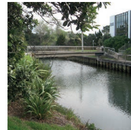
D. Existing pedestrian bridge. Orientation does not provide best connection to Beachfront Lane
