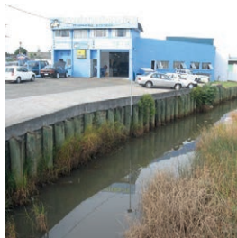
B. Veg type 3: Retaining wall and brackish wetland in stream. LID and stormwater treatment possibilities
