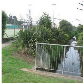
B. Exit from floodbank culvert, existing native vegetation but both banks are retained
