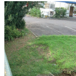
E. Consideration needed of treatment of culverts
