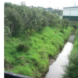
E. Retained bank to the right. Views from Glencoe Road to the left are restricted
